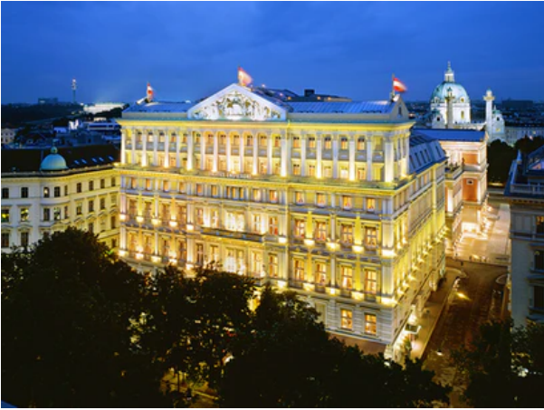
Photo courtesy of Hotel Imperial Save Place
